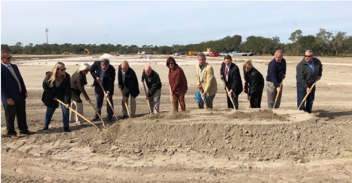
Scott Deal (tan coat, center), CEO of Maverick Boat Group in Fort Pierce, and members of the Economic Development Council of St. Lucie County and other officials celebrate the groundbreaking of a 106,000 square foot facility to build Cobia boats in Fort Pierce.
