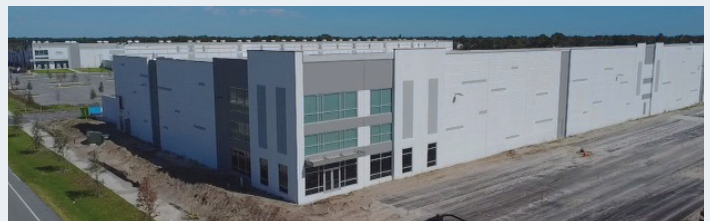
Legacy Park 168,000 SF industrial facility (Nov. 2022)
