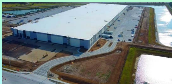
Kings Logistics Center construction was in the homestretch in May.
