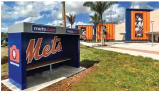
A $2.6 million renovation project was recently completed to replace the Clover Park baseball field in time for the New York Mets spring training.
