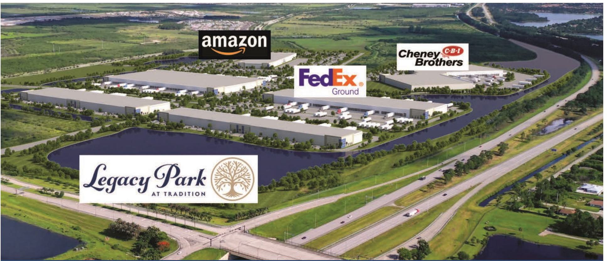
Legacy Park at Tradition, a 425-acre Class-A industrial park in Port St. Lucie, developed by the Sansone Group. Current tenants include Amazon and FedEx Ground, food distributor Cheney Brothers' warehouse is under construction, as are two spec buildings; build-to-suit locations are also available
